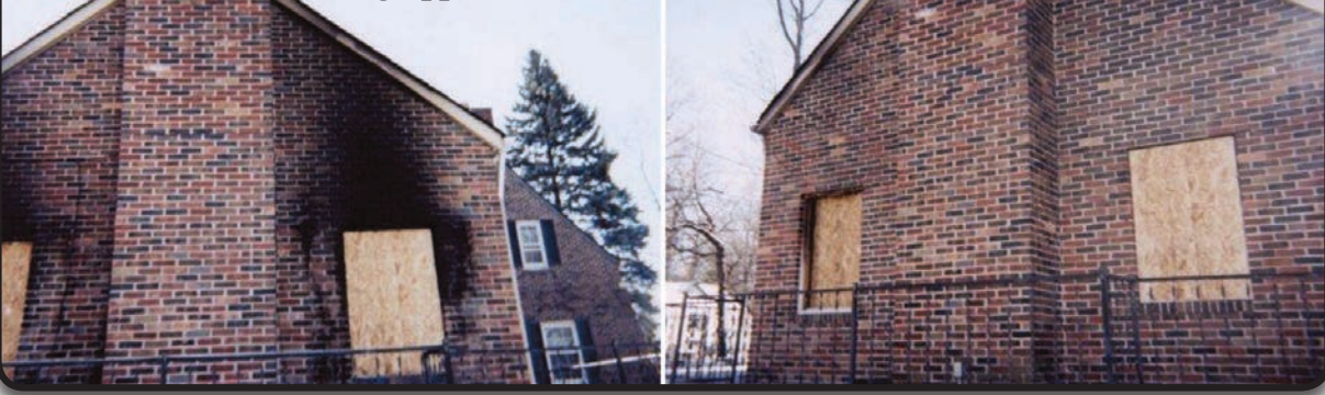
Fire Restoration Cleaning Applications
